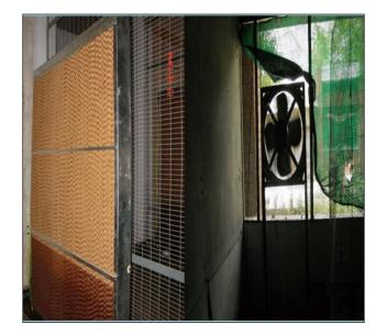
**Fig. 2:** The fan-pad system consisted of cellulose pads placed along the width-wise of the shed and the exhaust fan of 18" size fitted at the opposite end
